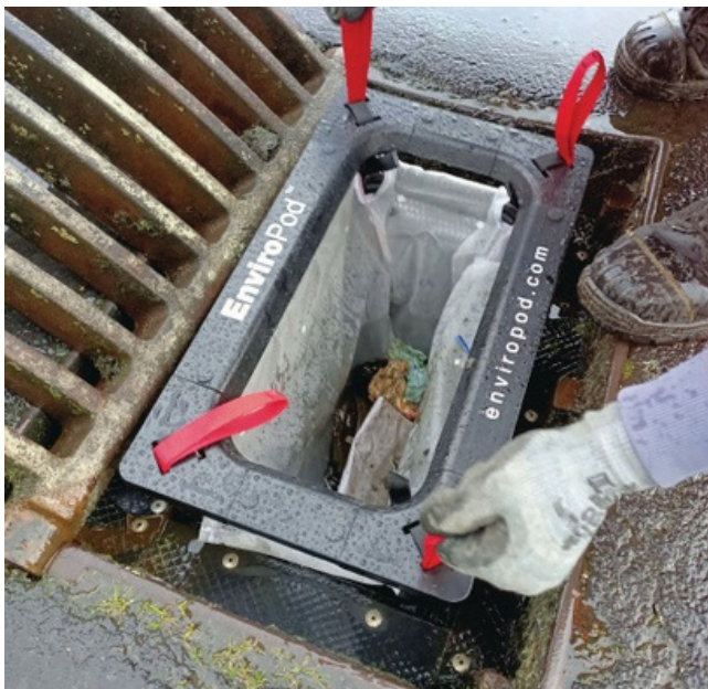
Figure 4: LittaTrap seen with 1mm liner installed to target micro-plastics such as plastic pellets. Hand maintenance shown.
