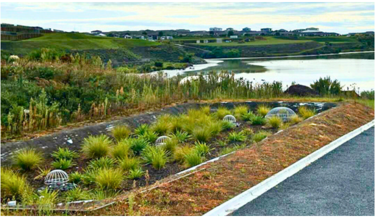
Ōmokoroa Filterra® Bioscape®: Catchment area: 3.25 hectares Bioscape® footprint: 120m²
