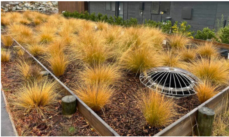
Lake Tekapo Filterra® Bioscape®: Catchment area: 5.1 hectares Bioscape® footprint: 165m²
