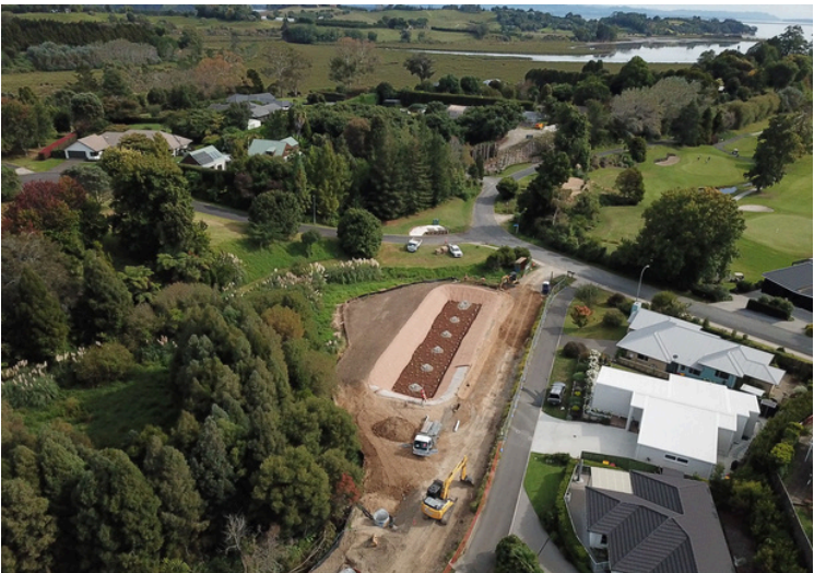
Ōmokoroa Filterra® Bioscape®: Catchment area: 5.6 hectares Bioscape® footprint: 205m²
