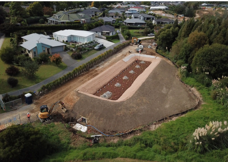
Ōmokoroa Filterra® Bioscape®: Catchment area: 5.6 hectares Bioscape® footprint: 205m²
